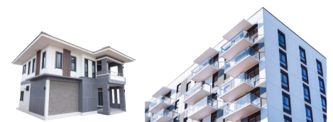
RESIDENTIAL AND COLLECTIVE INSTALLATIONS
